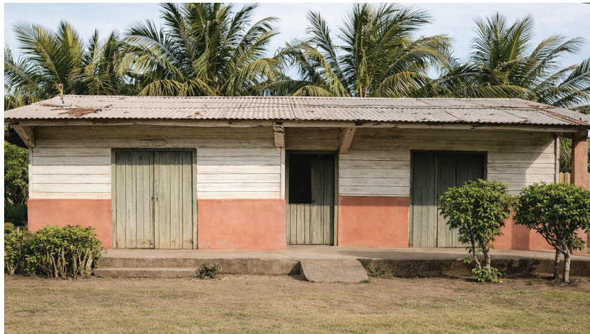
One of the current buildings of the Centre, Photo. M. Ochlak OMI
